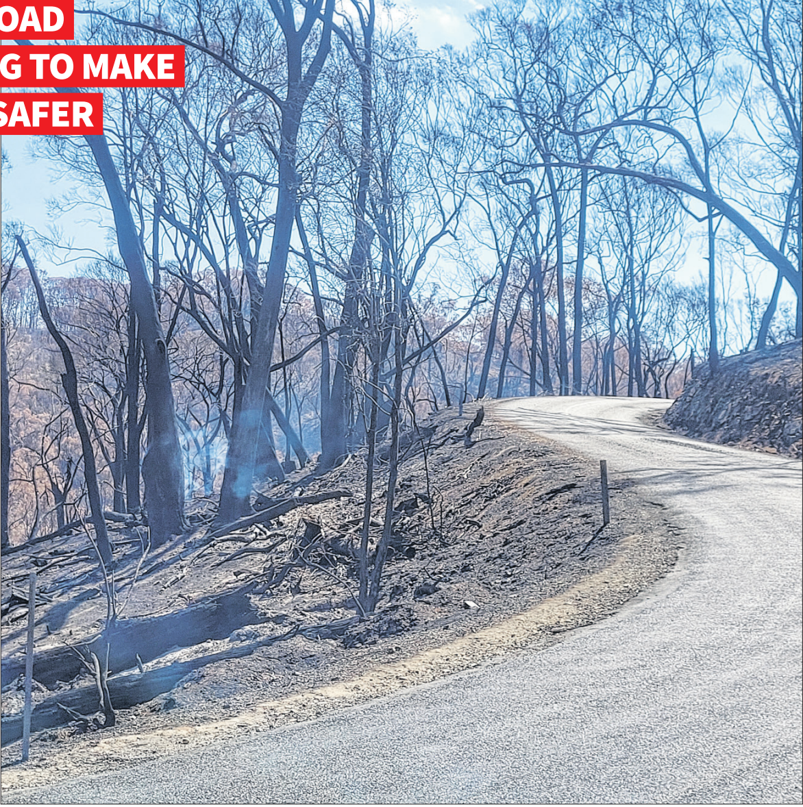
ROAD SAFETY THE PRIORITY: The ‘Gobur Cutting’ on Yarck-Gobur Road after the Longwood fire, when the trees were still smouldering. The petition is calling for funding to make this section of road safer. PHOTO: Bailey Dixon
