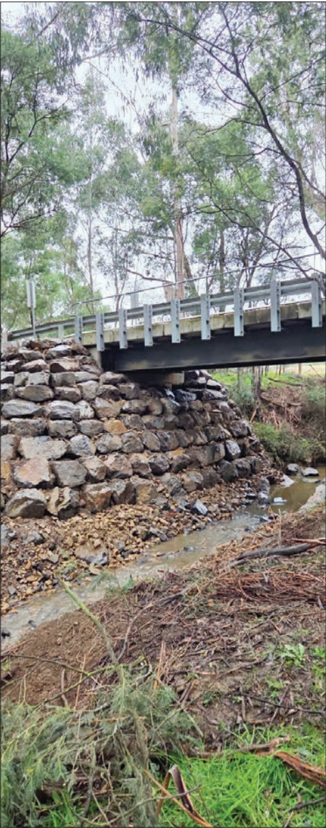
BUILDING BACK BETTER: Walls Road Bridge in Glenburn after the restoration works were completed.
