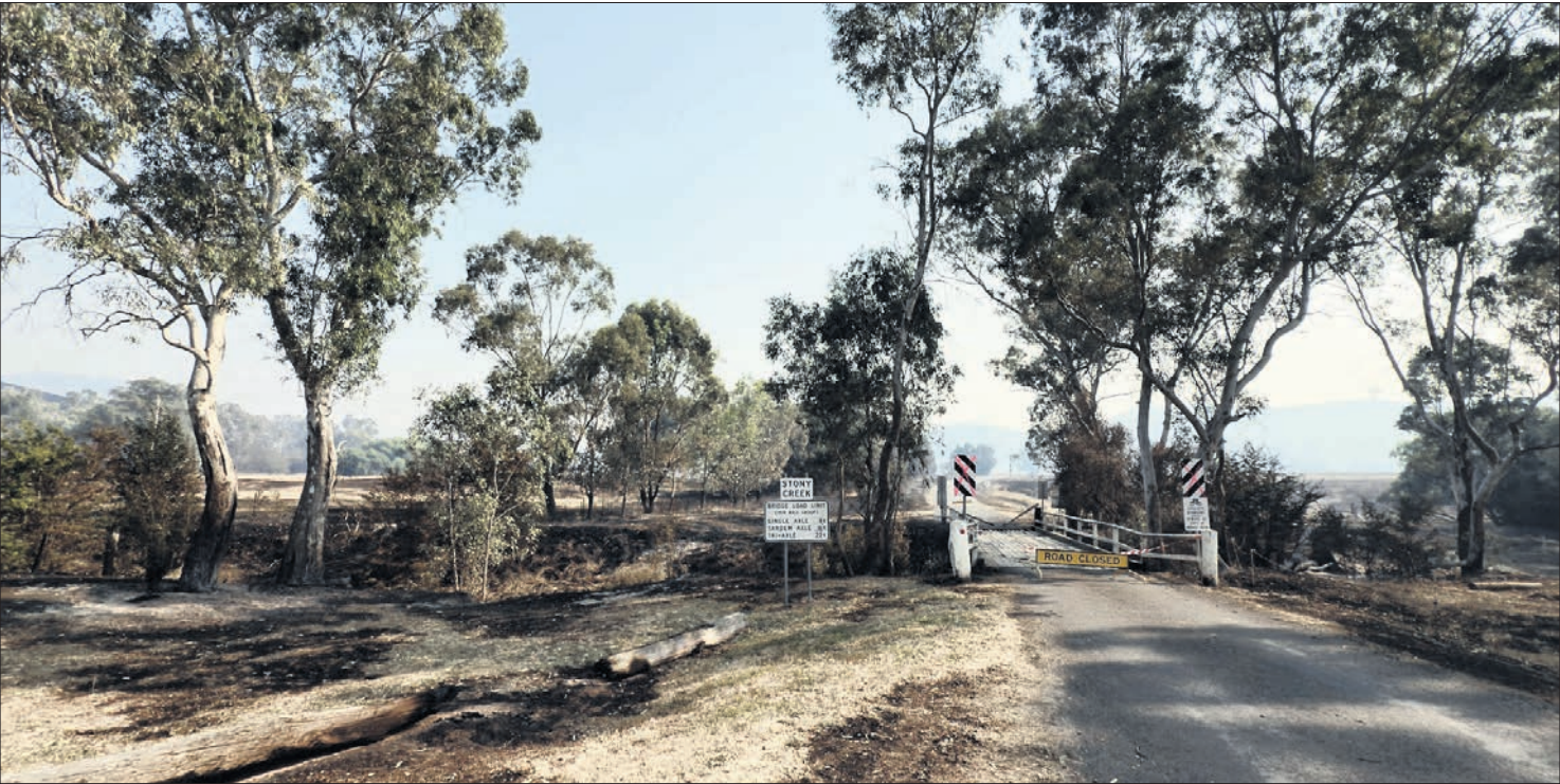
BRIDGE MENTIONED IN PARLIAMENT: The fire-damaged Fawcett bridge.
