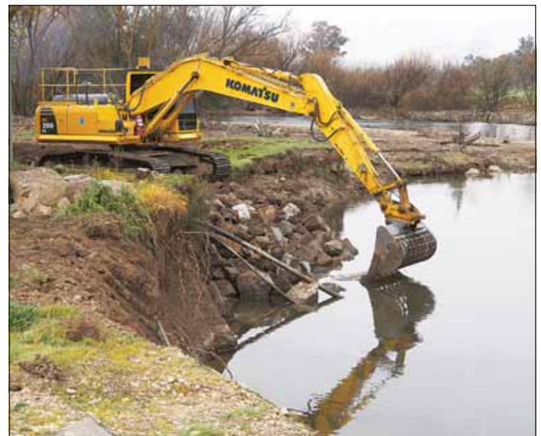
Filling the left side embankment. -AR
