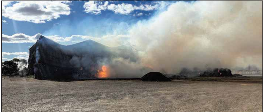
Hay bale fires can lead to a lot of damage. This was a large shed for storing hay. -S
