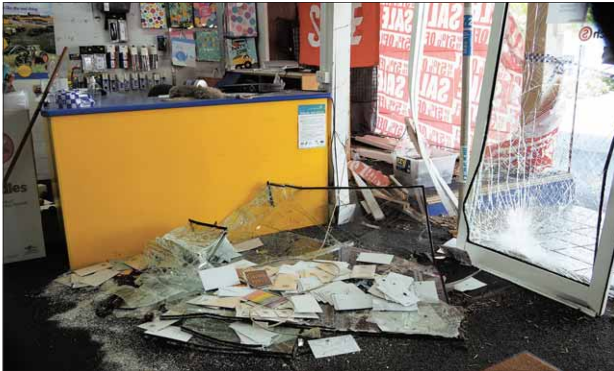
The damage inside the store following the incident. -AR
