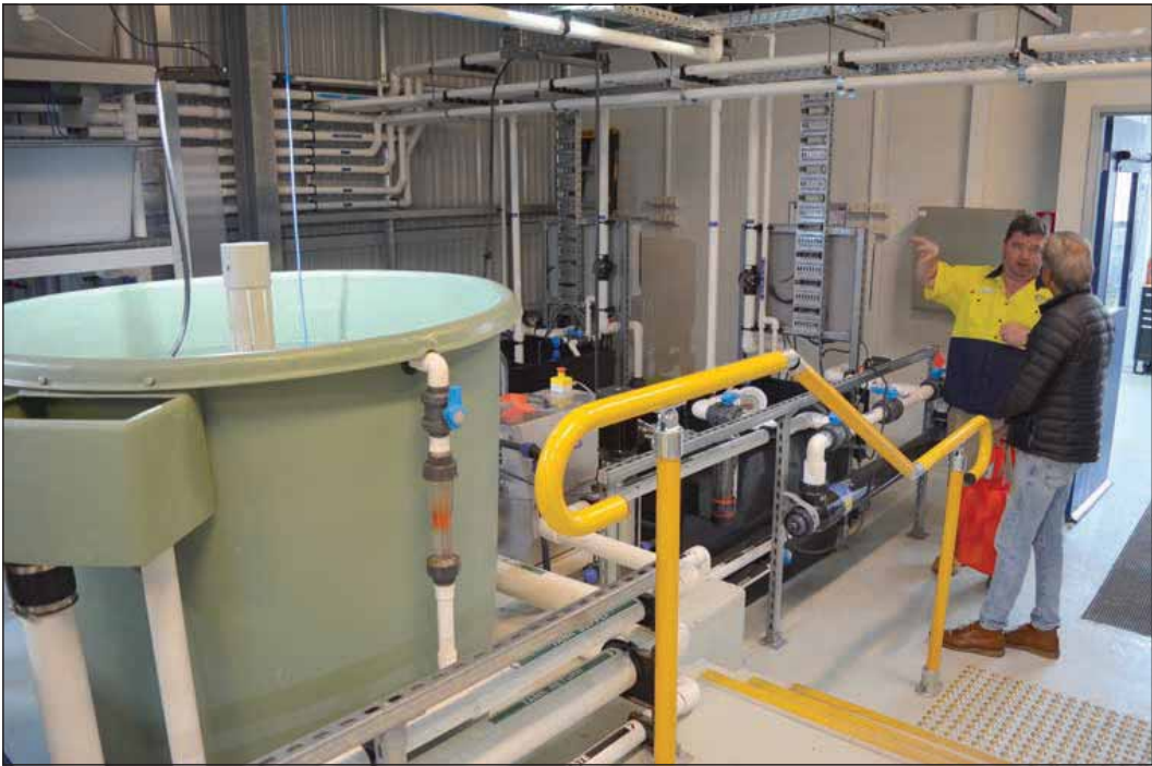
One of the tanks in the conservation hatchery and its filtration system. -BD
