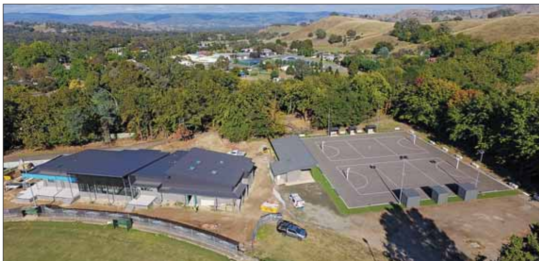
Works near completion but with more to go. - S
