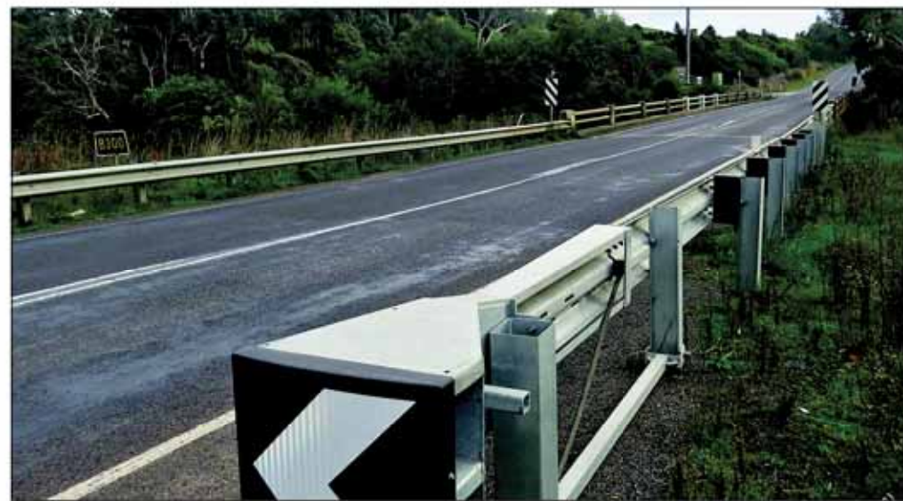
Devlin's Bridge. -S
