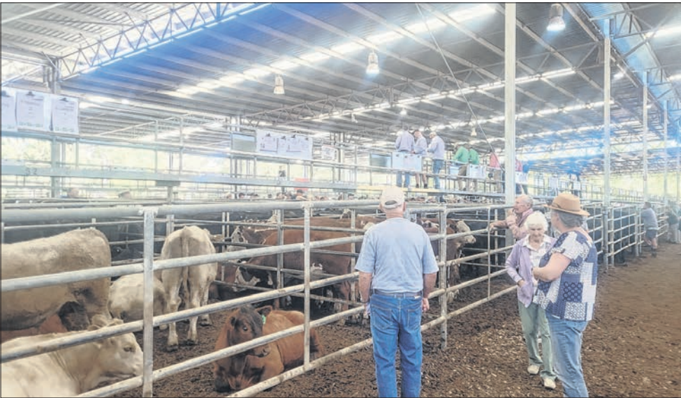
BUILDING FOR THE FUTURE: Yea Saleyards has received a grant to install an integrated solar, battery and generator-backed power system at the Yea Saleyards. PHOTO: Bailey Dixon
