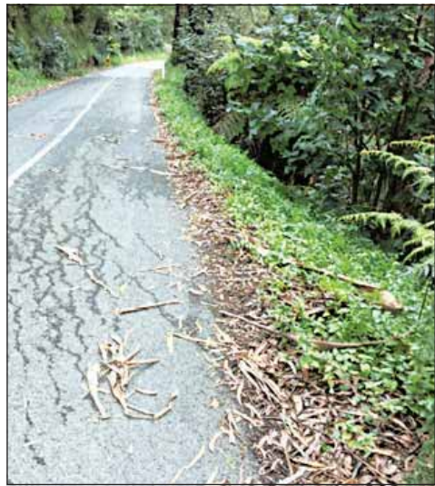
Castella Road with damage to road seal, following the October 2022 flood and storm events. -S
