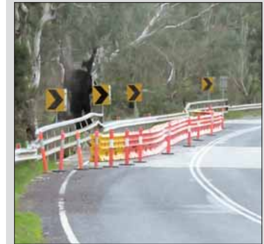
The Dairy Creek Bridge. -S
